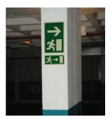
Standard rectangular Type 1 signs often do not suit installation onto pillars due to their shape and a reduced effective viewing distance due to their relative size. Evacuation signs specifically developed for pillars allow pictograms to be larger, therefore providing a greater viewing distance. The image shown illustrates the comparison between the two types of evacuation signs and the pictogram size.
