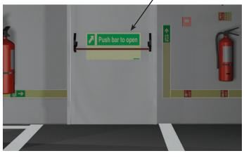
The emergency exit opens on the right hand side and this is indicated by the signs and strips being positioned to the right and parallel to the door opening mechanism.
