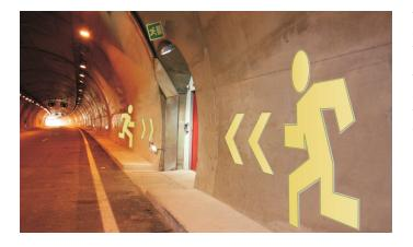
The installation of large signs in close proximity to an emergency exist will allow the exit to be identified more readily and will therefore minimise the risk of panic.
