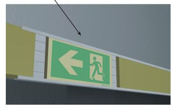
A sign indicating the direction of the evacuation route is positioned in between two strips which, in the example, have been installed with a vandal-proof aluminium rail.
